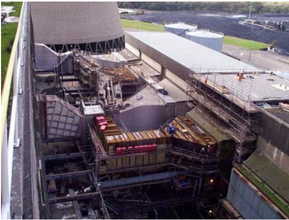
Typical Rebuild of an existing Electrostatic Precipitator
